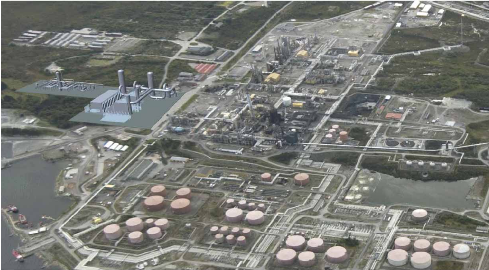
Fluor Daniel Econamine FGSM Retrofit at a gas-processing plant.
