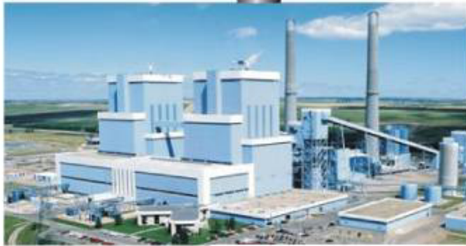
Antelope Valley Station
