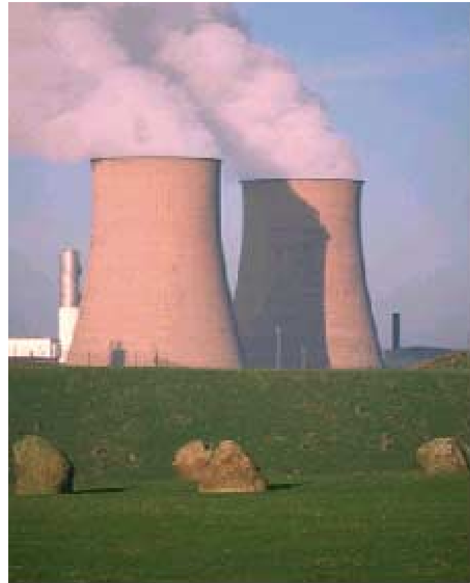
Power Plant Cooling Towers
