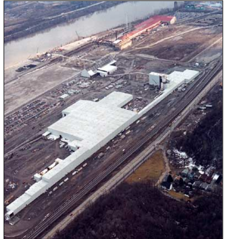
USG Wallboard Plant, Aliquippa, PA
