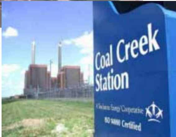
Great River Energy's Coal Creek Station, North Dakota
