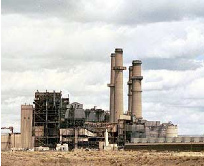
San Juan Generating Station
