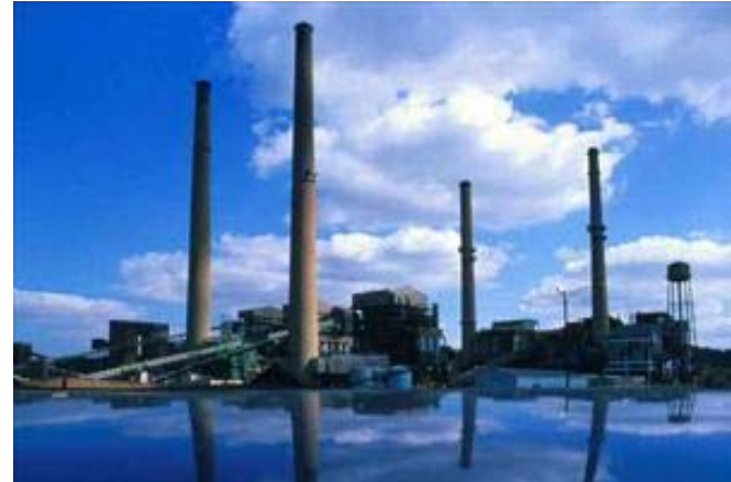
Conesville Power Plant, Coshocton, OH
