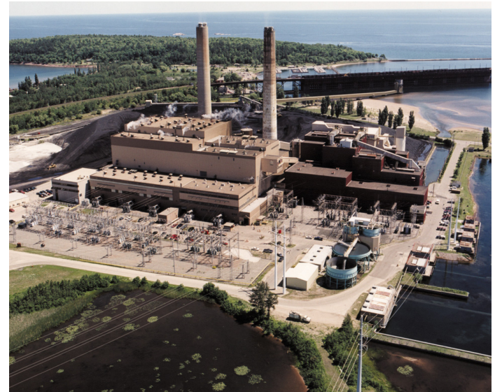
We Energies Presque Isle Power Plant
