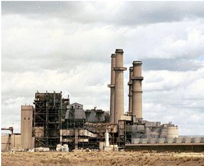
San Juan Generating Station
