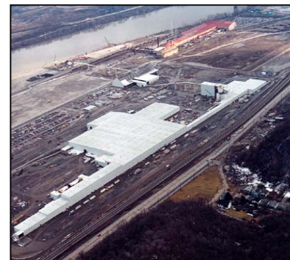
USG Plant, Aliquippa, PA
