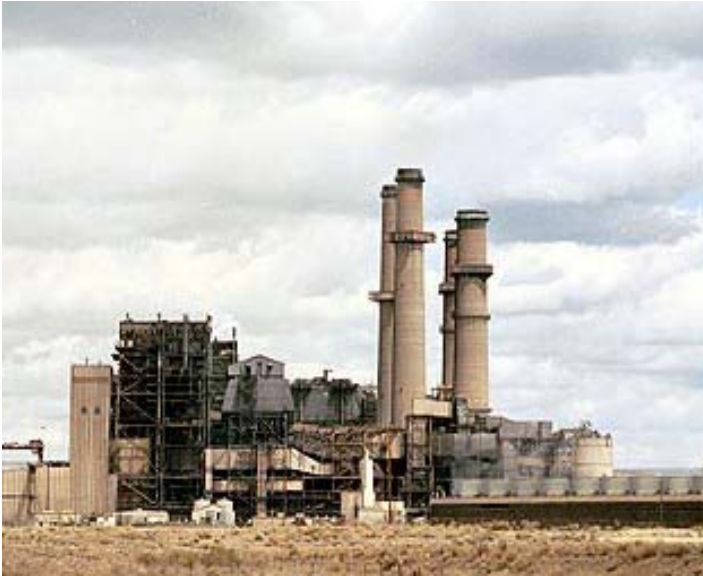
San Juan Generating Station
