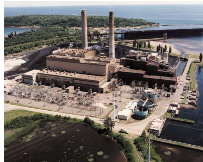
We Energies Presque Isle Power Plant
