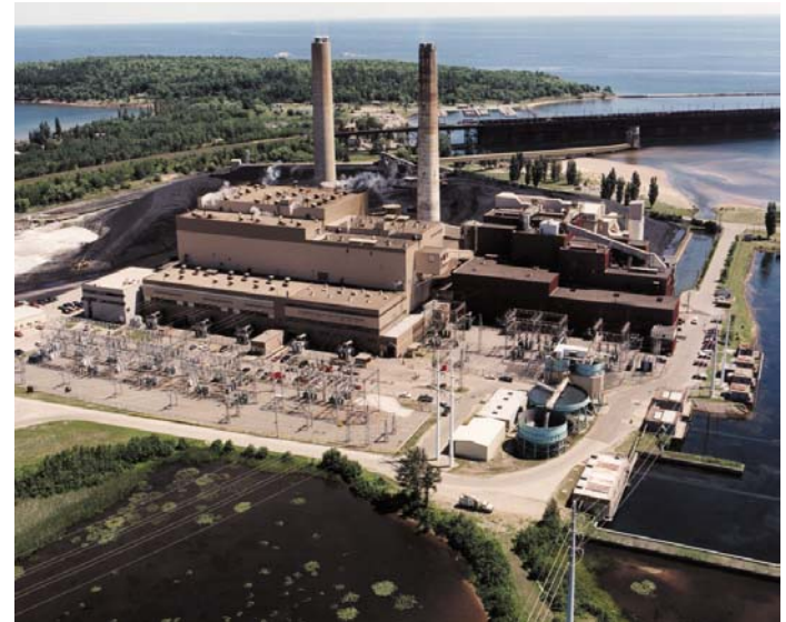
We Energies Presque Isle Power Plant
