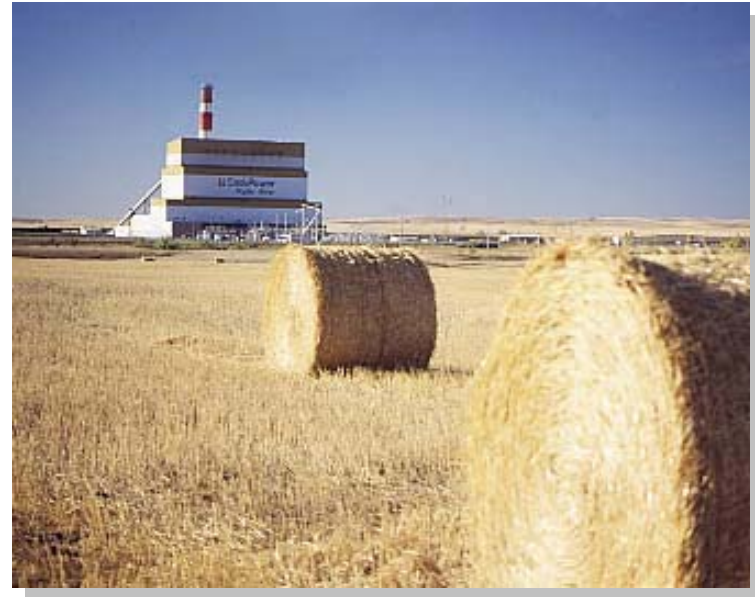
SaskPower's 562-MW Lignite-Fired Poplar River Power Plant
