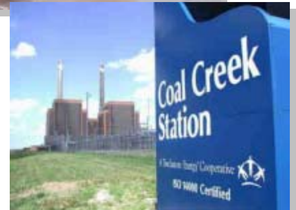
Great River Energy's Coal Creek Station, North Dakota
