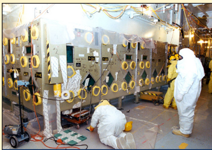
Gloveboxes prior to chemical decontamination at Rocky Flats.
