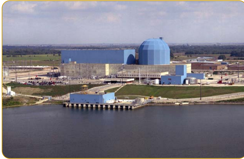
Clinton Nuclear Power Station at the Exelon Clinton site in Illinois
