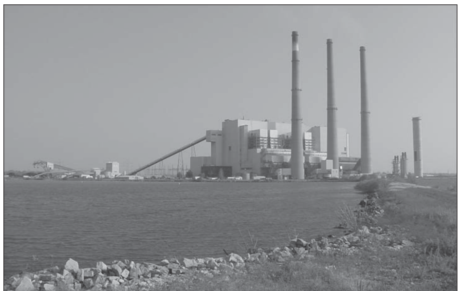
Advanced optimization software for enhanced emissions control is being demonstrated at Dynegy Midwest Generation's Baldwin Energy Complex in Baldwin, Illinois.
