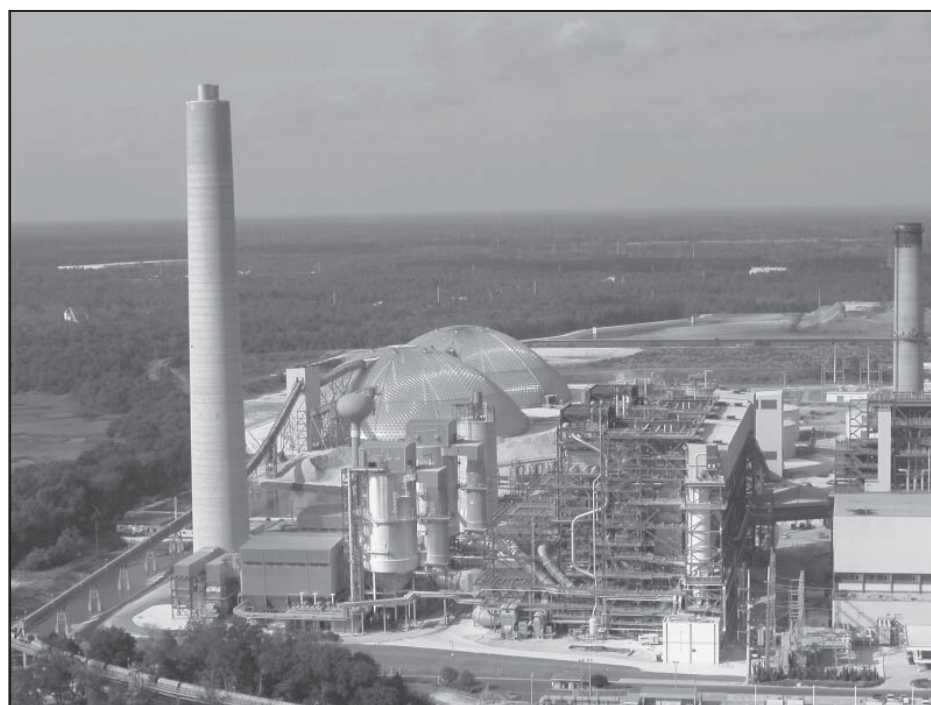
Advanced CFB is being demonstrated at JEA's Northside Station in Jacksonville, Florida.
