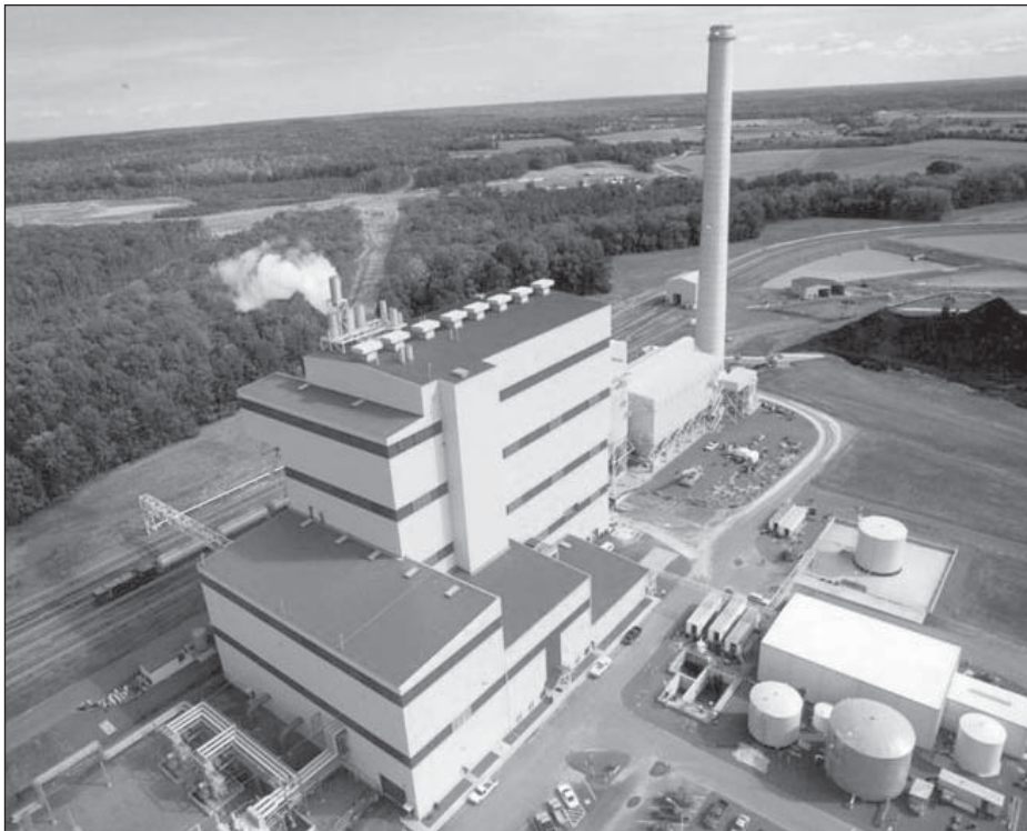
Conversion of spray dryer ash to lightweight aggregate for construction materials is being demonstrated at the Birchwood Power Facility in King George, Virginia.
