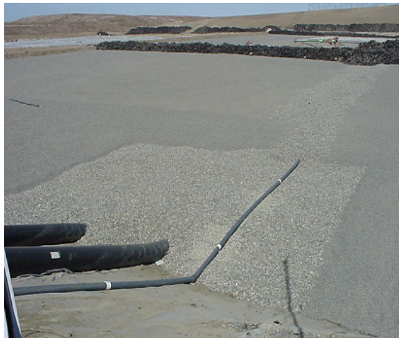
Waste Containment Base Liner System
