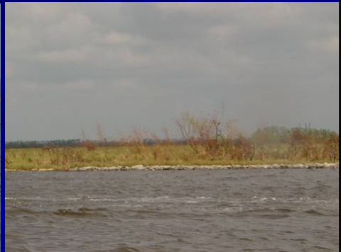
No shoreline erosion due to Hurricanes Katrina and Rita – protection feature part of Jonathan Davis Wetland Project (BA-20).
