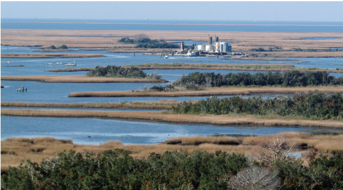
Figure 3. Threatened Port Facility
