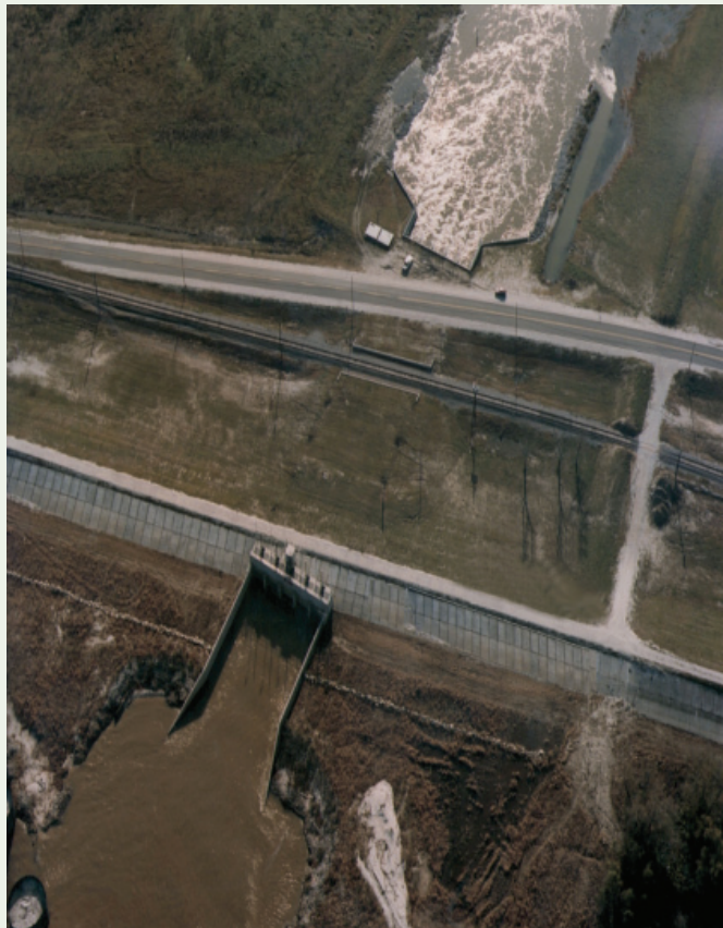
Caernarvon Freshwater Diversion Structure
