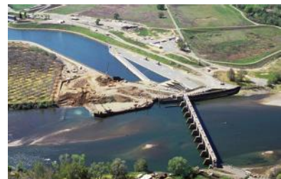
Red Bluff Diversion Dam
