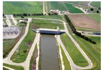
Formerly referred to as the Tracy Pumping Plant, it was renamed in 2006 to the C.W. "Bill" Jones Pumping Plant
