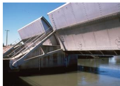
Fresh water from the Sacramento River comes through the Delta Cross Channel Gates into the Delta's interior
