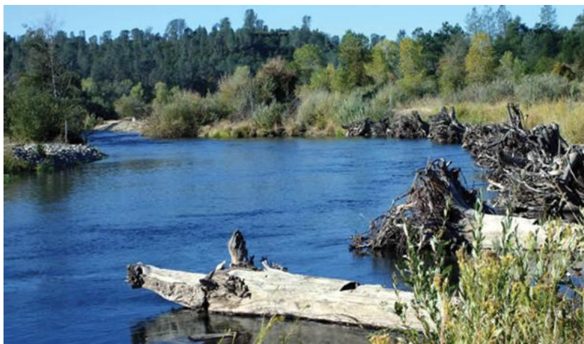
Anchored root balls of large trees help keep the Creek in the desired channel
