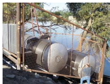
RD 999's cylindrical screen on the Sacramento River
