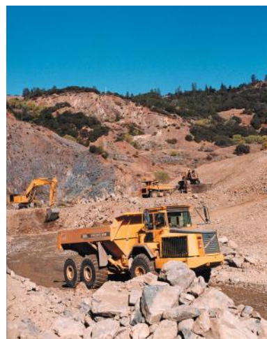
Construction activities at the American River Pump Station
