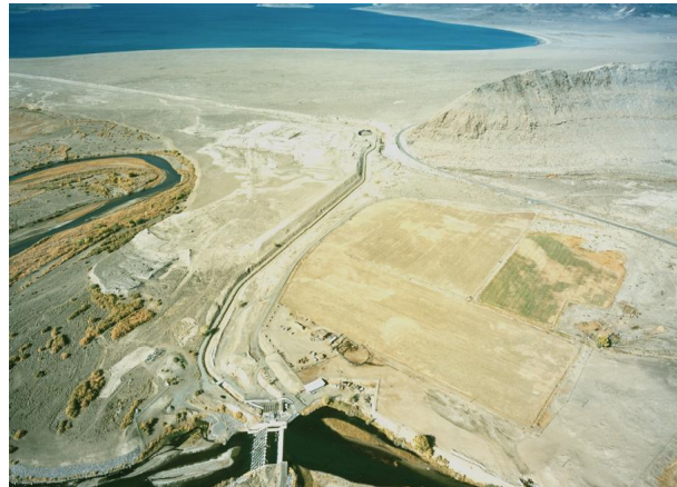
Marble Bluff Dam on the lower Truckee River
