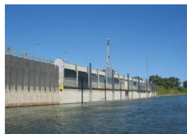
Reclamation District 108's new fish screen at Wilkins Slough
