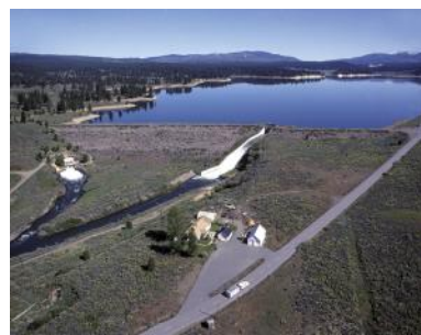
Boca Dam and Reservoir, part of the Truckee River Storage Project
