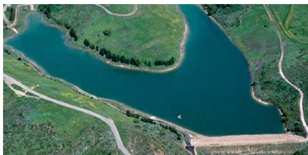
Lauro Dam aerial view
