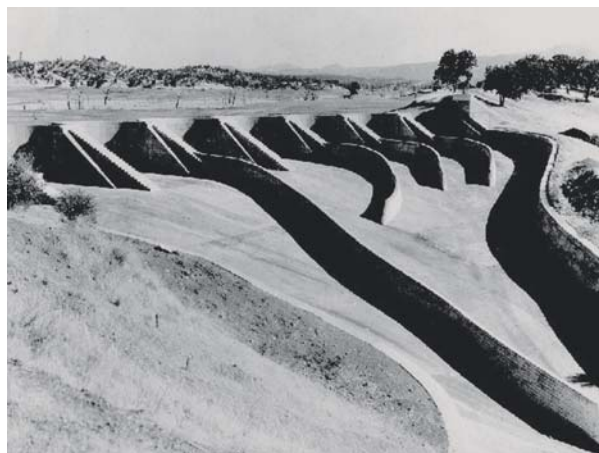
East Park Dam spillway
