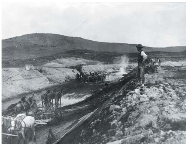
Excavating a Canal in Klamath Falls, Oregon - 1906
