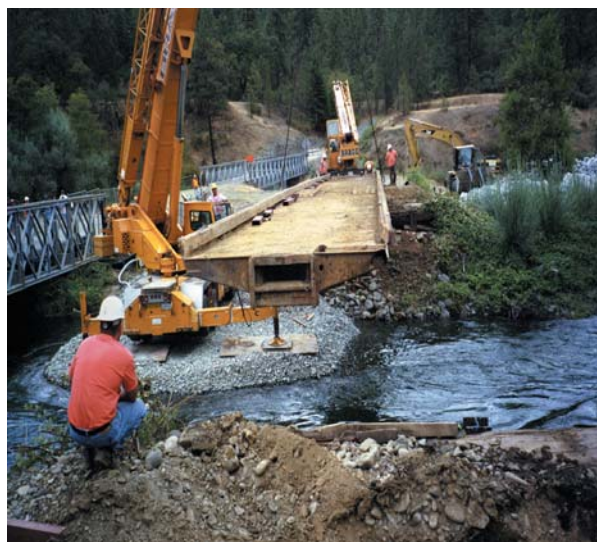
Trinity River bridge construction under way in 2005.
