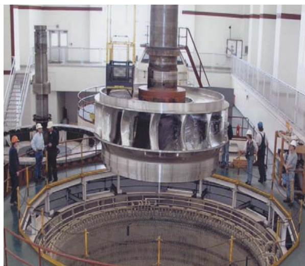
Turbine runner replacement at Shasta Powerplant
