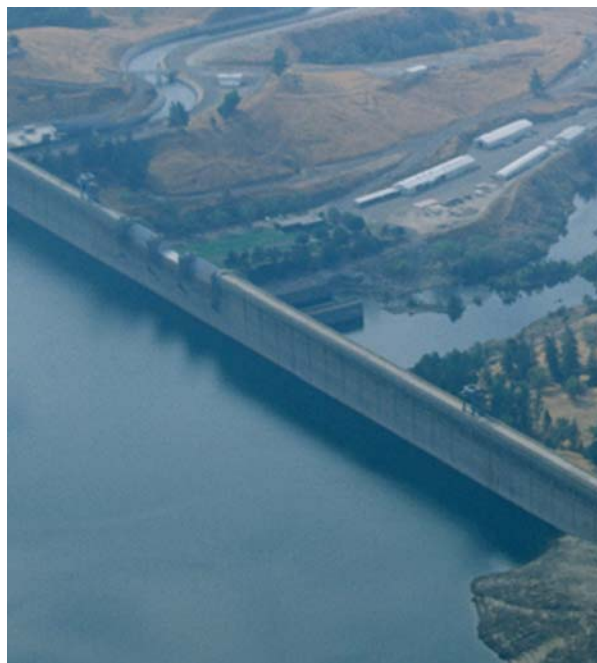
Aerial rear view of Friant Dam
