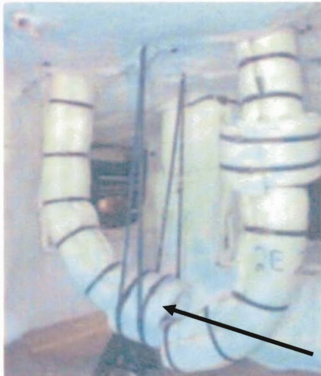
Post Fire Test (Note Change in Color of Outer Wrap)
