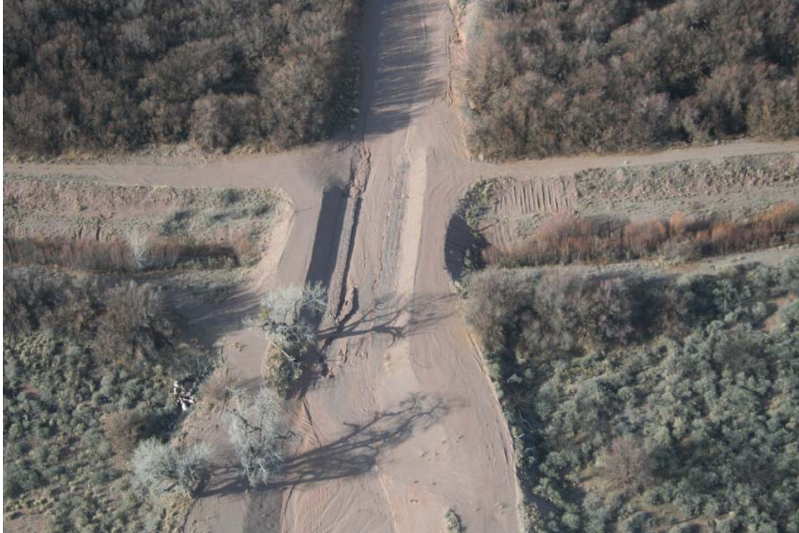
Photo 3. Completed Phase I work on Escondida Drain at Arroyo de los Pinos. Taken facing east (January 2008).
