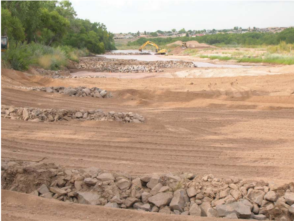
Photo 8. Installation of bendway weirs at the Sandia priority site (September 2007).
