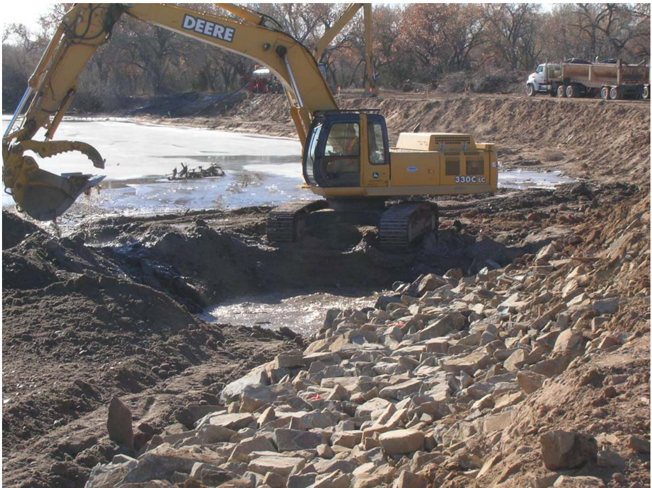
Photo 5. Installation of a riprap toe on the bankline at River Mile 231.3 (January 2008).
