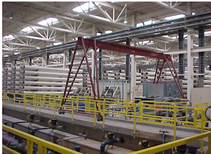
Figure 3-3.—YDP Crane Assembly for Removing Pressure Vessels
