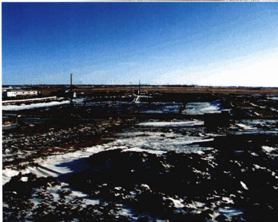
Figure 4.—Installation of FT intake structure.
