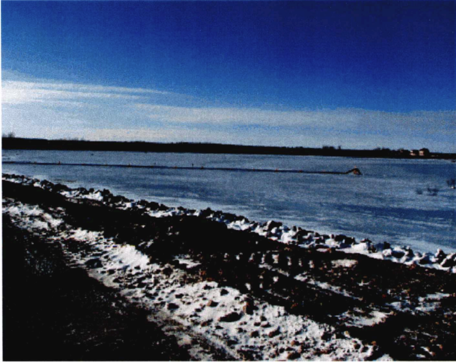
Figure 7.—FP1 upright sprays and piping.
