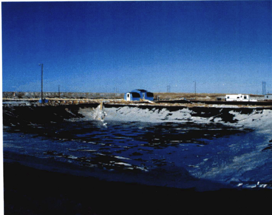
Figure 3.—HDPE liner in brine pond.
