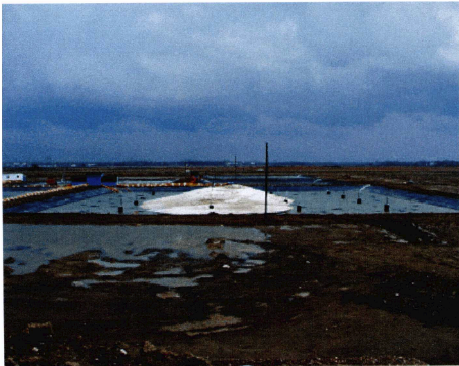
Figure 13.—FP1 ice pile condition (April).
