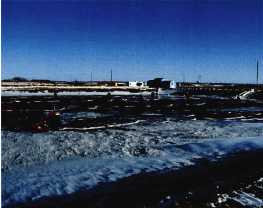
Figure 5.—FT feed line after installation.
