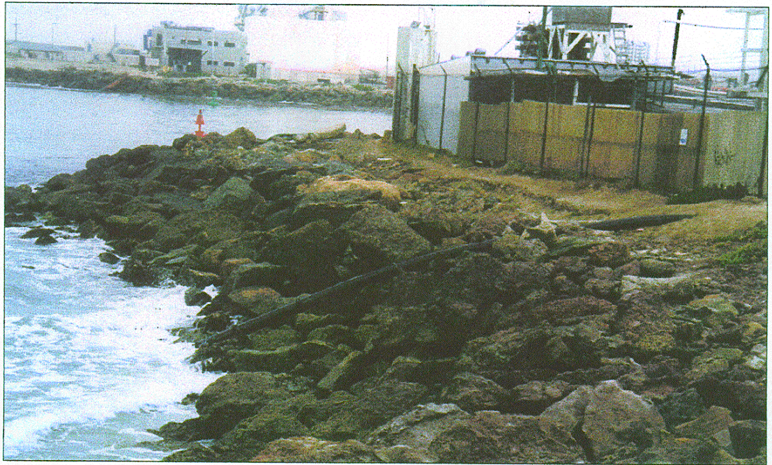
Figure 10a. SWISS Intake Piping.
