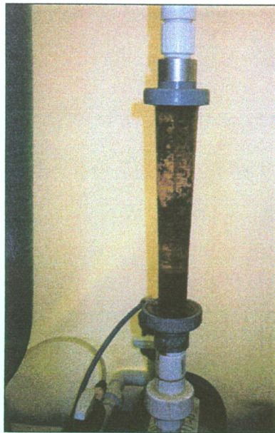
Figure 14-a. Open Water Intake Flowmeter.
