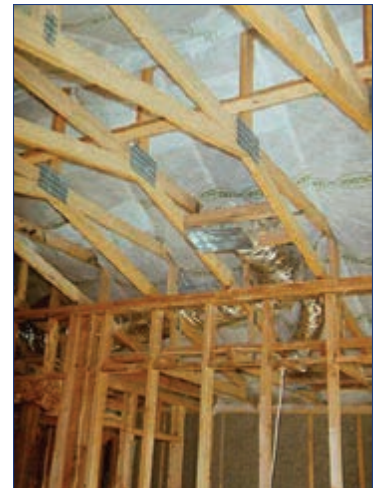
Careful attention went into sealing and insulating the attic.
