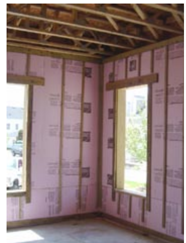
FIGURE10: Masonry Walls with Interior Rigid Insulation
