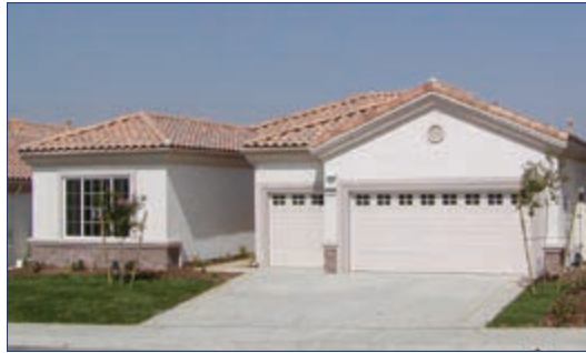
Using innovative construction methods and Building America know-how, Pulte built 600 homes in its Sun Lakes development in Banning, California, all of them 15% to 20% over California's new Title 24 requirements.
