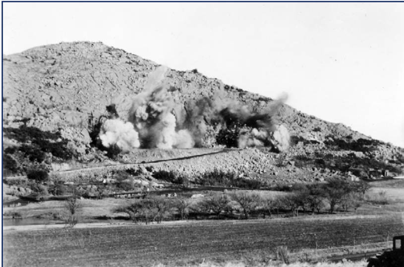
First telephoto shot of large blast of the rock quarry used to supply the granite for the construction of Altus Dam, December 16, 1940.
