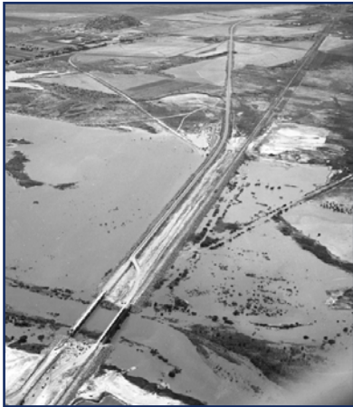
View of ongoing reconstruction of Oklahoma State Highway No. 9 bridge across the upper end of Lake Altus, July 7, 1947 (National Archives and Records Administration 1947b). The earthen approaches of this bridge constrict the lake and have effectively separated the reservoir into two pools, one upstream (right) and one downstream (left) of the crossing.
