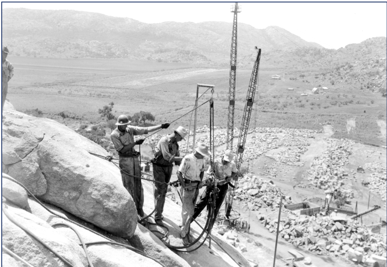
Drilling crew at work on rock face of mountain above quarry bench, July 9, 1941. Below, granite blocks are separated by size and shape for use as facing or riprap in the construction of Altus Dam (National Archives and Records Administration 1941a).
