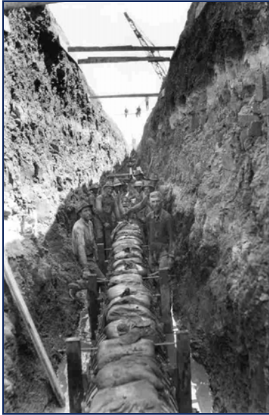
Construction of the redwood pipeline that carried water from the original Lake Altus Dam south to the city of Altus, circa 1927. Photo courtesy of the Museum of the Western Prairie, Altus, Oklahoma. Used with permission.
