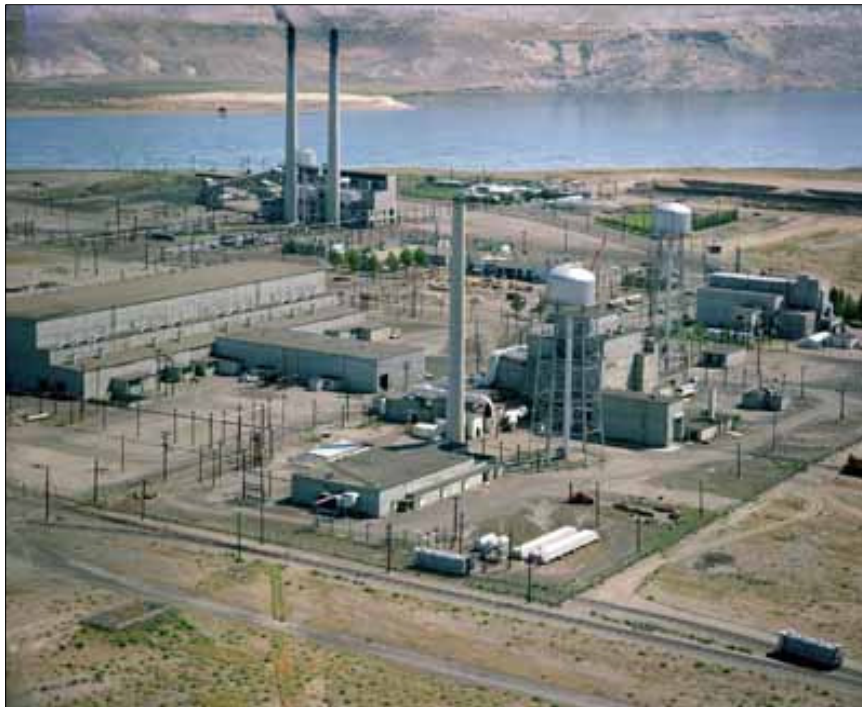
Hanford's F Reactor – completely dismantled in 2003
