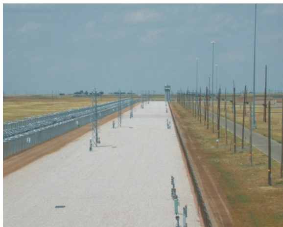
PIDAS (Perimeter Intrusion Detection Access System).
