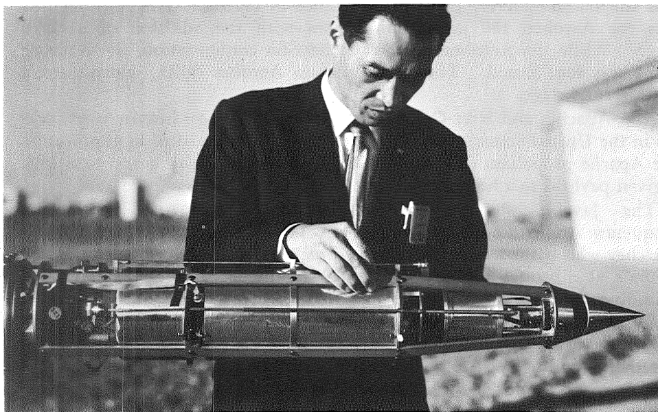
A closeup of the sounding rocket used in the first joint flight effort by the United States and Japan being checked by a Japanese scientist.
