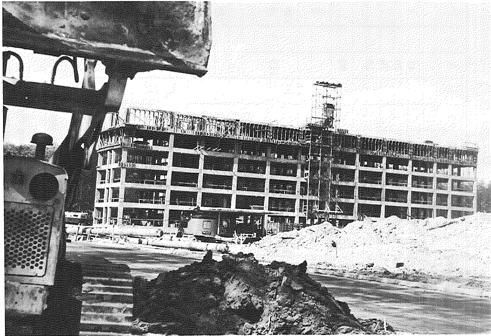
Building 8 under construction, July 1962.
