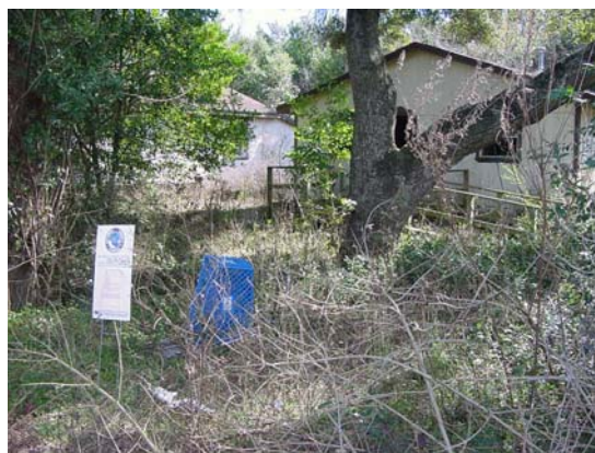
A condemned property near the Escambia site (EPA OIG photo)
