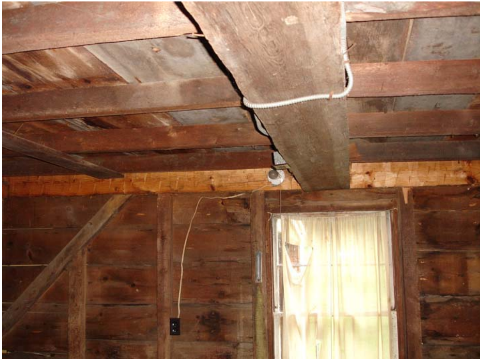
Figure 62. Elisha Jones Shed: Shed Room 104, east wall, exposed framing including summer beam, 1974 replacement girt, studding, and bracing (2006).
