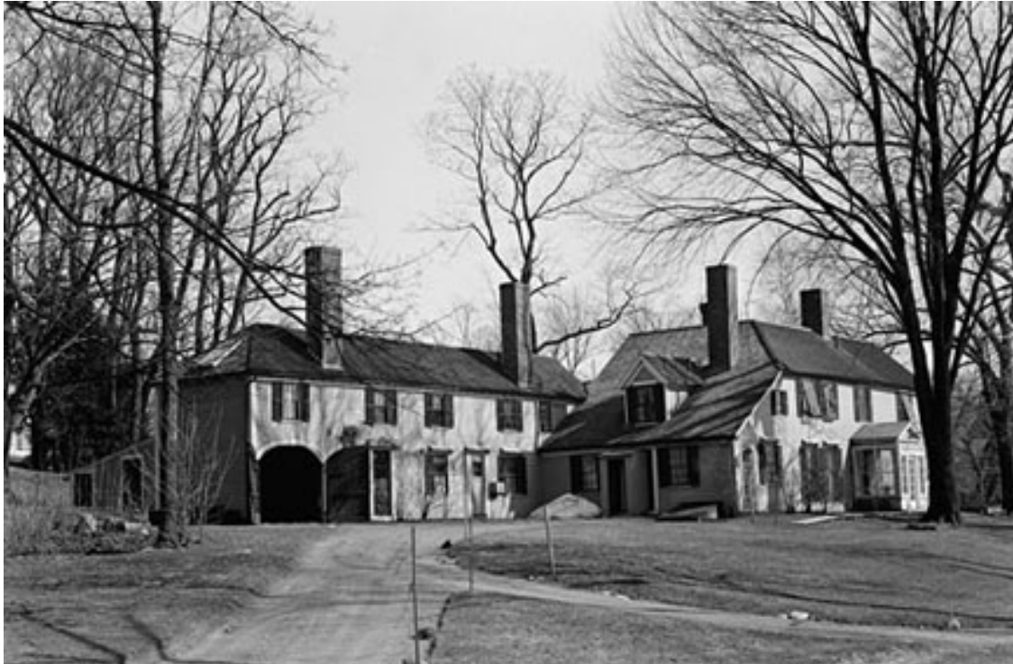
Figure 28. Elisha Jones House and Shed: North and west elevations, April 7, 1941.
