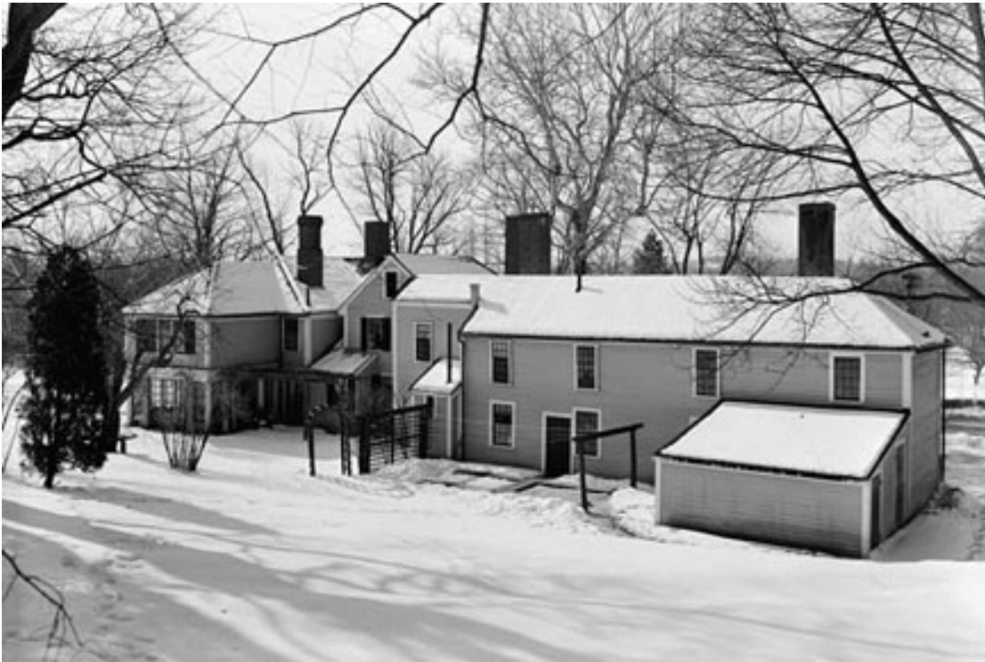
Figure 30. Elisha Jones House and Shed: East elevation, February 1963.
