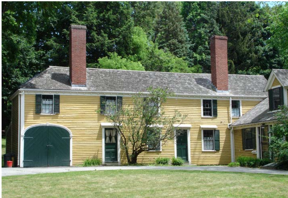
Figure 4. Elisha Jones Shed: West elevation.
