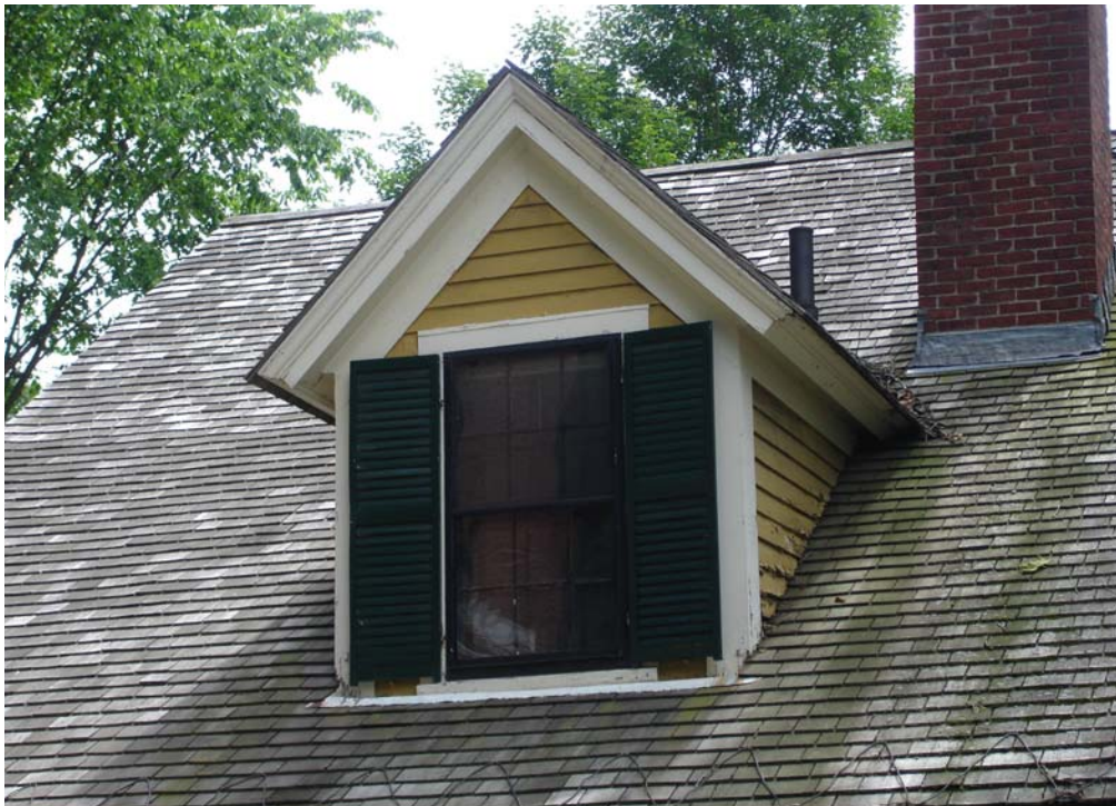
Figure 27. Elisha Jones House: Dormer on north roof (2006).
