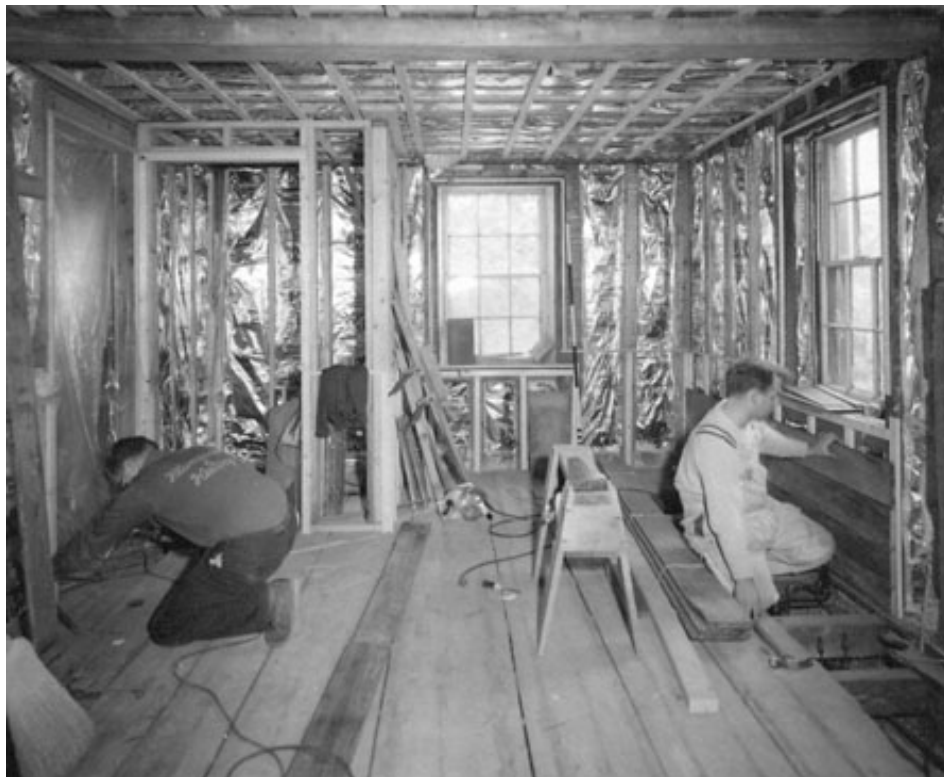
Figure 33. Elisha Jones House: East extension of north lean- to, installation of chestnut wainscoting in kitchen ell during 1966 rehabilitation work.
