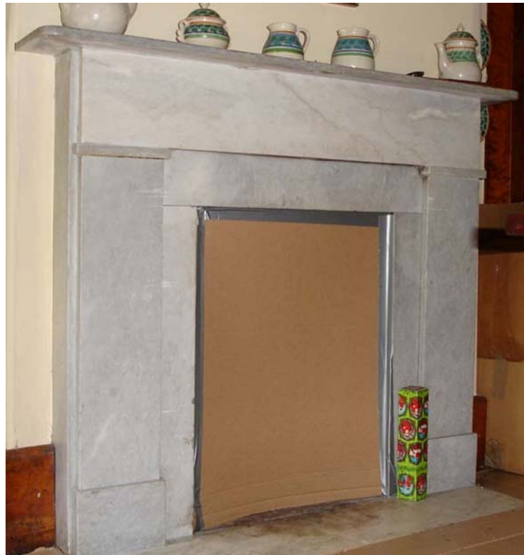
Figure 53. Elisha Jones House: Study (Room 104), marble fireplace surround and mantelshef (2006).
