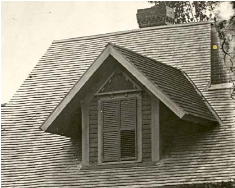
Figure 26. Elisha Jones House: Dormer on north roof, ca. 1890.
