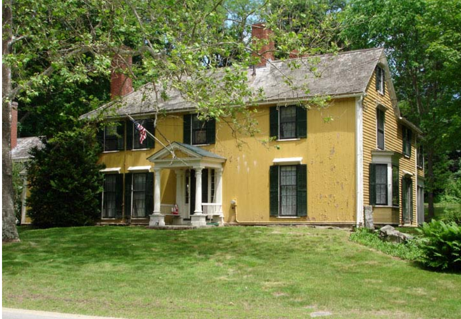
Figure 3. Elisha Jones House: West elevation.
