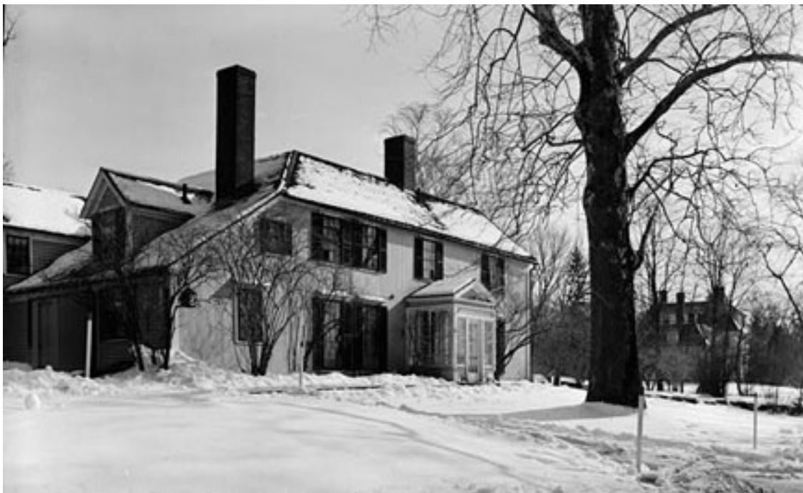
Figure 29. Elisha Jones House: West and north elevations, February 1963.
