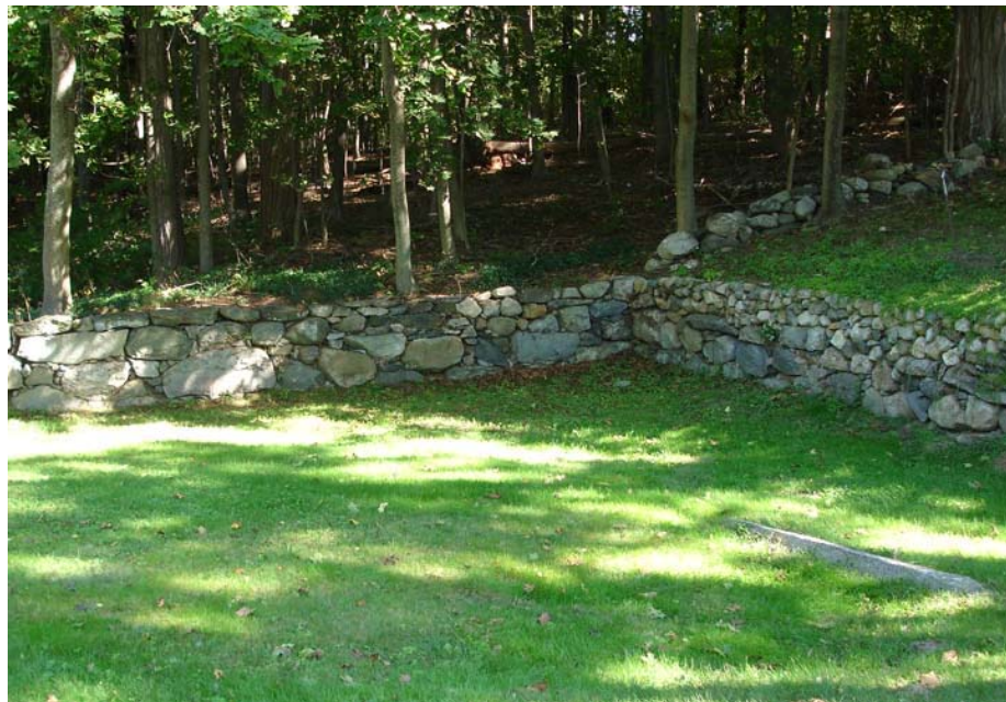
Figure 6. Keyes Barn foundation at Elisha Jones House.
