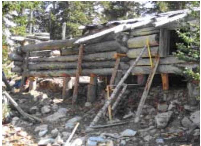
Photo 2. Cabin is stabilized after rotted logs have been removed.
