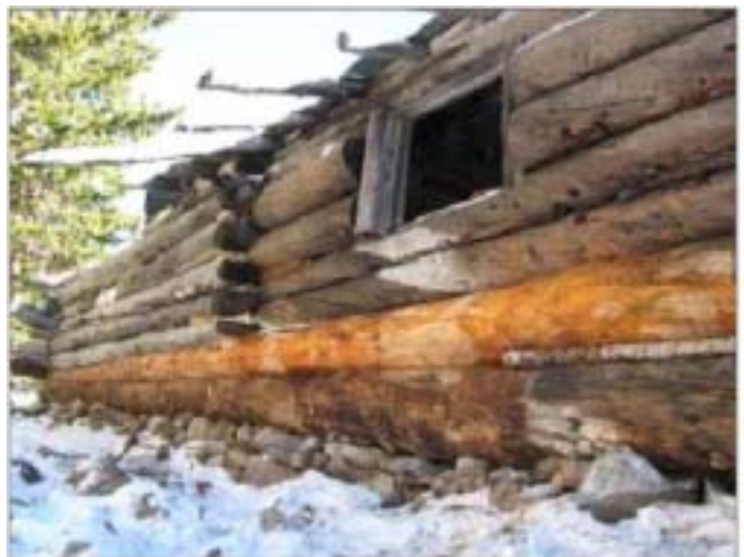
Photo 3. Cabin has new logs to help support and preserve it. Rocks are placed under the logs instead of soil to prevent decay.
