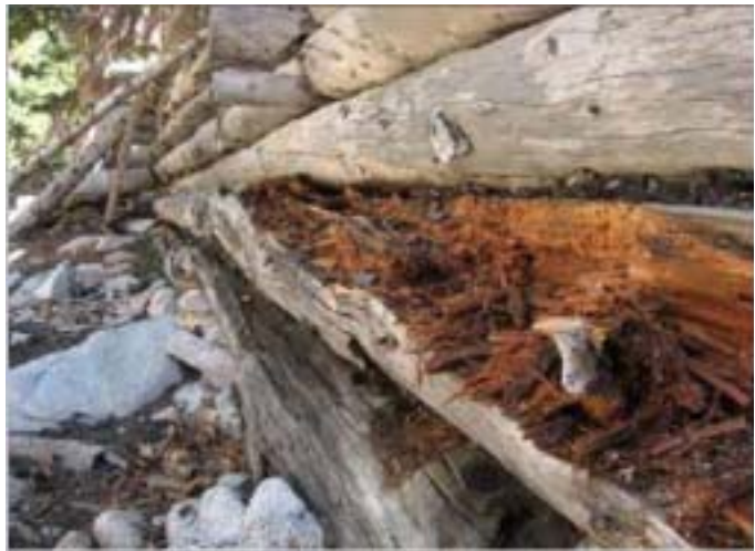
Photo 1. Logs at bottom of cabin were rotting.
