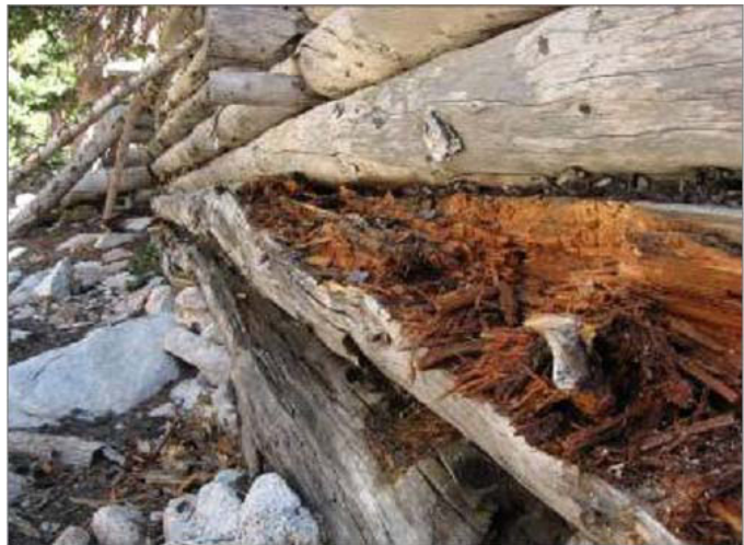
Photo 1. Logs at bottom of cabin were rotting.
