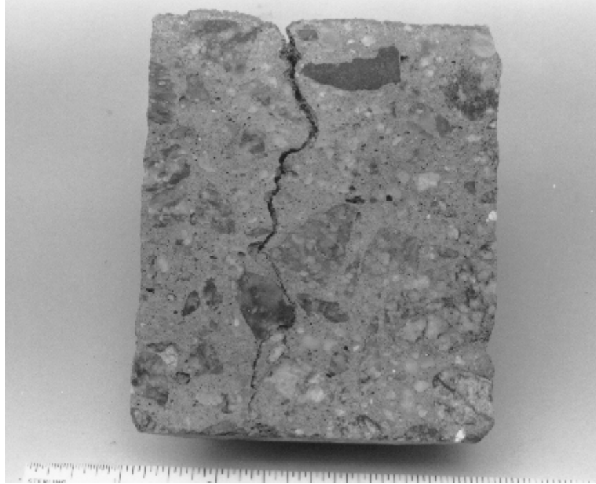
Figure 40. Plastic shrinkage crack on a lapped surface (wearing surface is at the top of the photograph).
