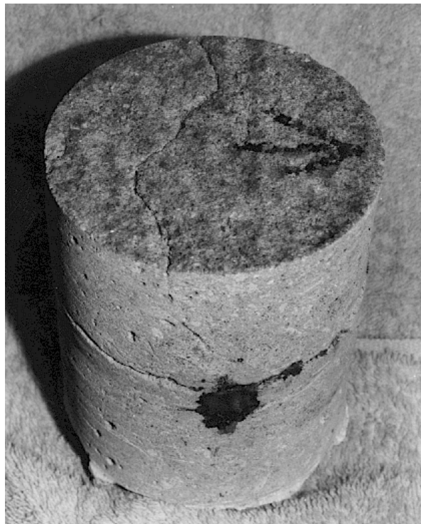
Figure 28. Cracking on surface and side of core with associated corrosion and expansion of the reinforcing bar.
