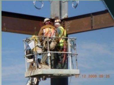
Welding Inspection
