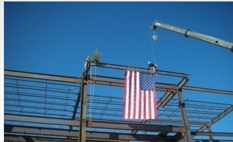
Steel Erection "Topping Out" (Fir tree symbolizes "Safe Completion")
