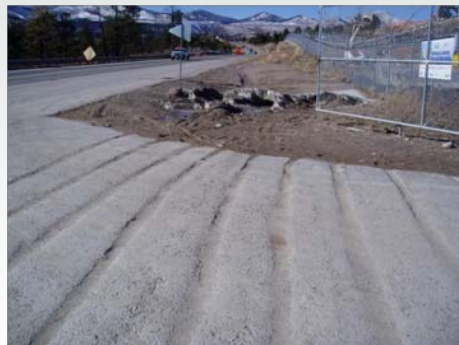
Grizzly track-out at construction vehicle access & egress for sediment transport control.
