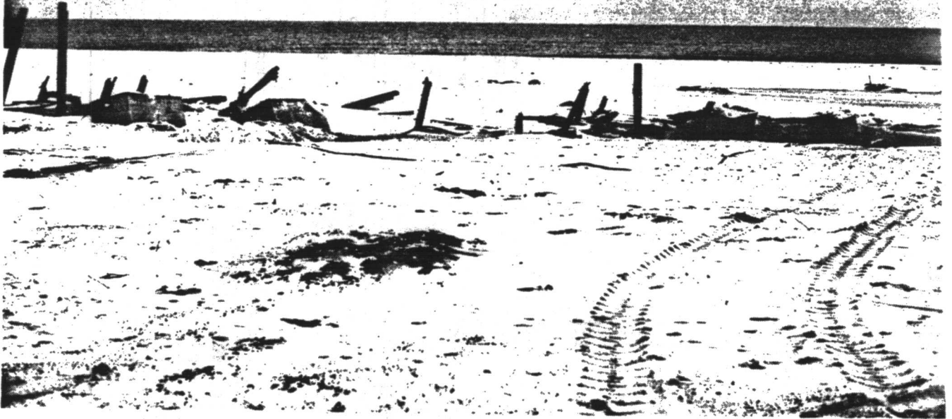
FIGURE 4a Septic tanks exposed by storm surge action of hurricane FREDERIC (1979) near Gulf Shores, Alabama (Courtesy of L. Handley).
