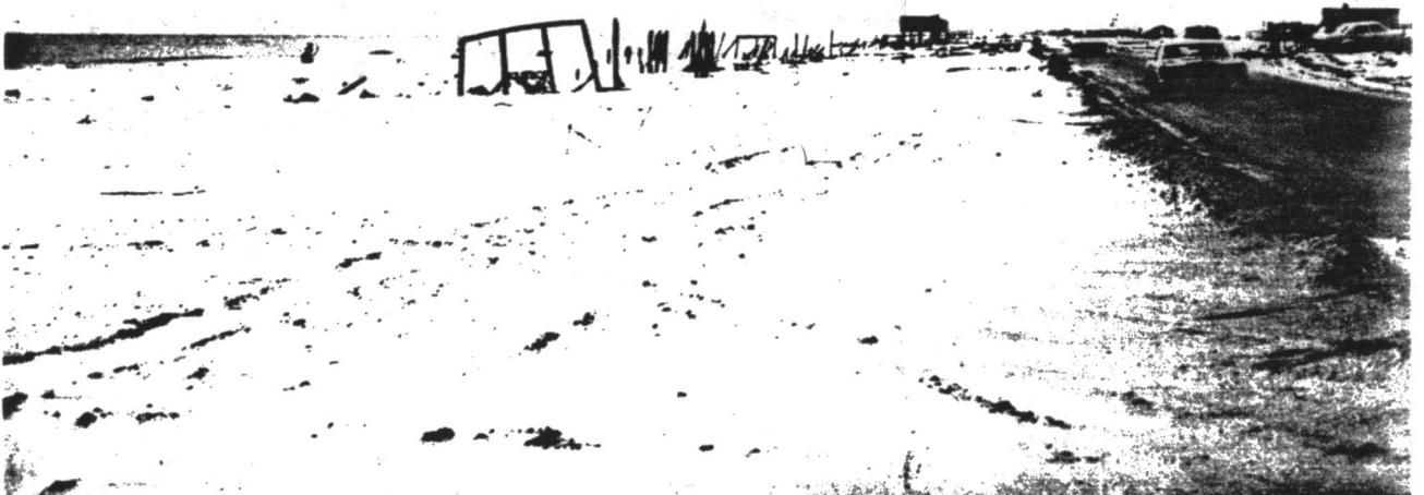
FIGURE 4b Following hurricane FREDERIC (1979) only pilings remain of houses that once stood near Gulf Shores, Alabama (Courtesy of L. Handley).
