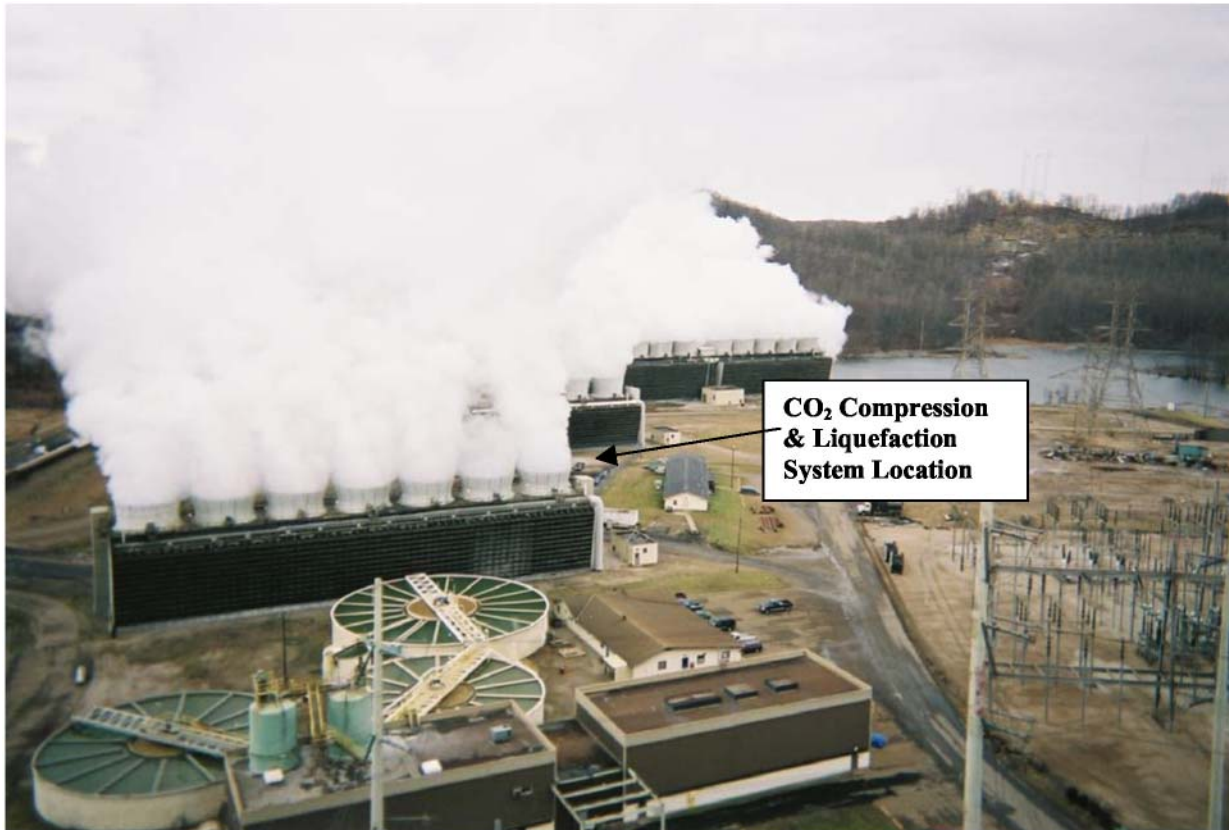
Figure 3-17: Existing Conesville Cooling Towers & CO 2 Compression/Liquefaction System Location
