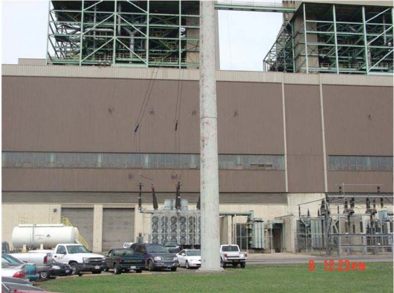
Figure 3-15: Conesville Unit #5 Existing Turbine Building
