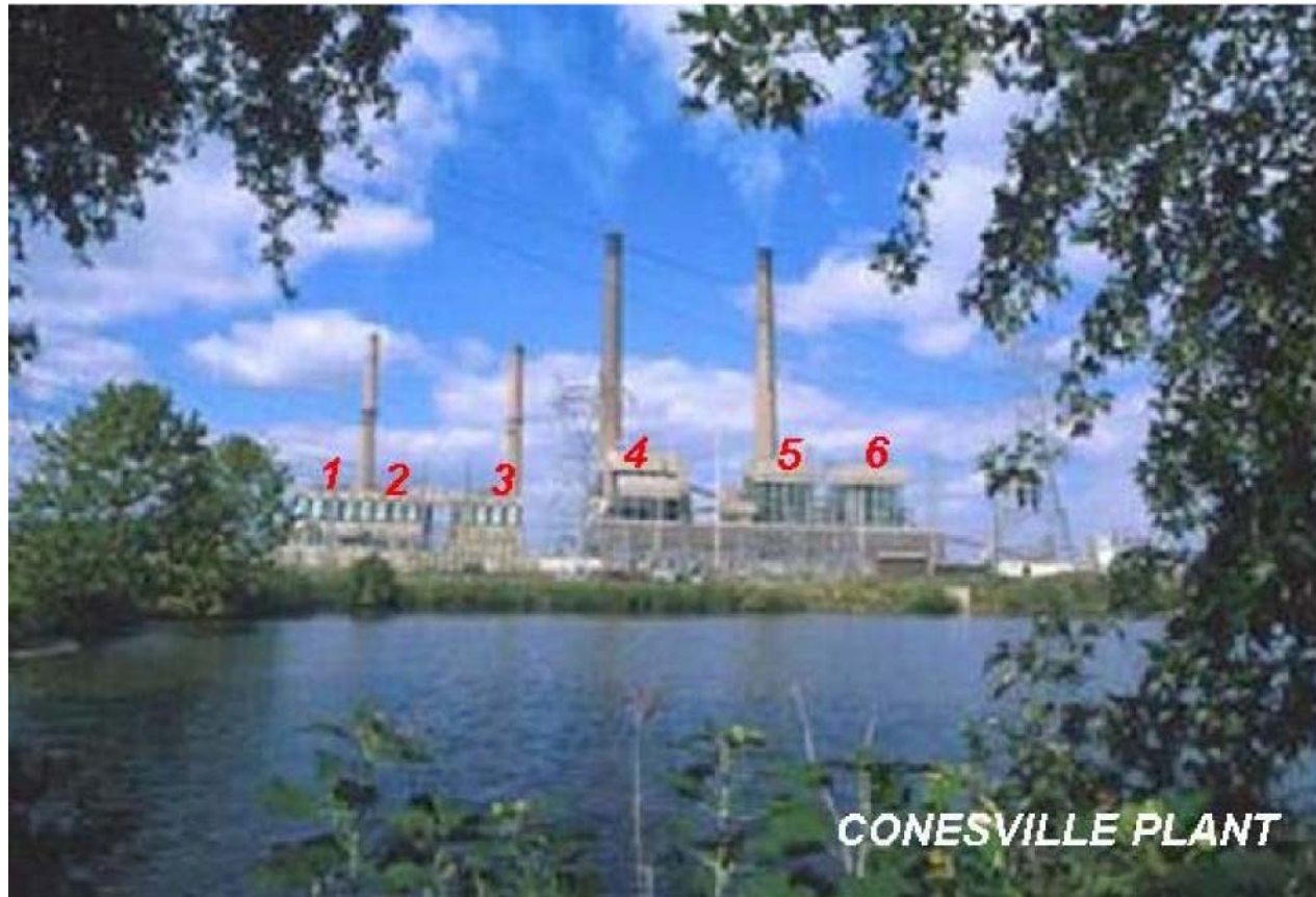
Figure 2-1: Conesville Power Station
