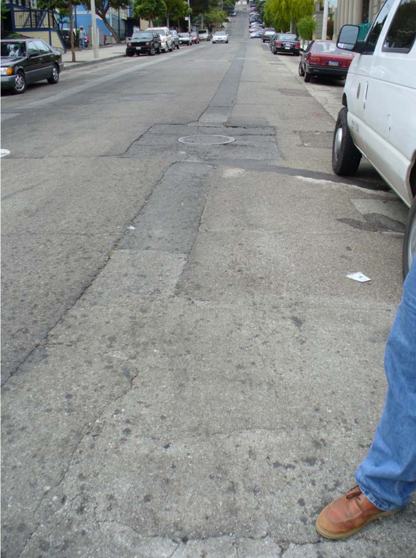
Figure 8: MTA Conduit Under Street With Electric Trolley Line
