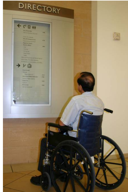
Figure: Building Directory that can be read from wheelchair
