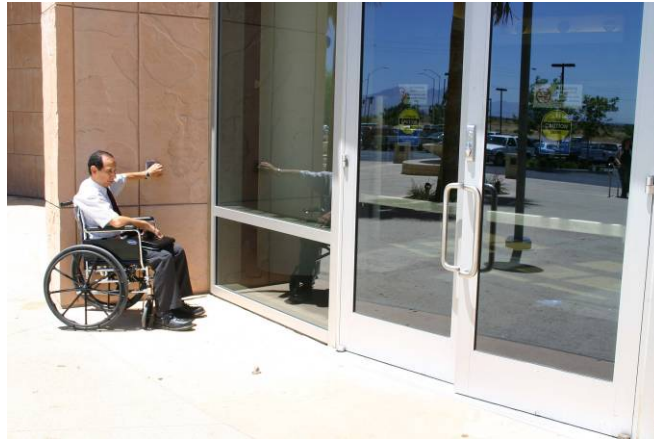
Figure: Exterior door with power operated door in use.
