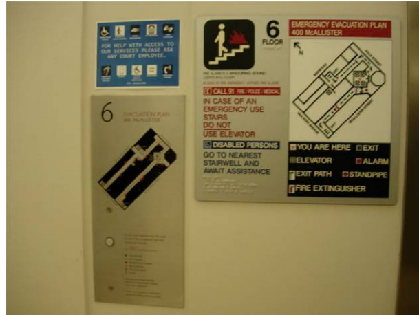
Figure: Signage next to elevators with directions for emergency evacuation. Avoid overly complicated signage
