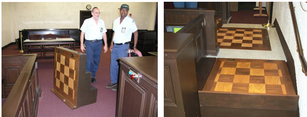
Figures: Common Error - The lift in the above courtroom requires the addition of a platform covering the stairs to be operable.
