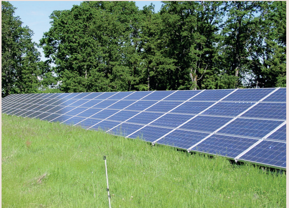
The solar electric systems at Raintree Tropical is comprised of 132 modules and is expected to save 25,000kW of electricity per year. Photo credit: Ann Grim, Oregon Department of Energy.
