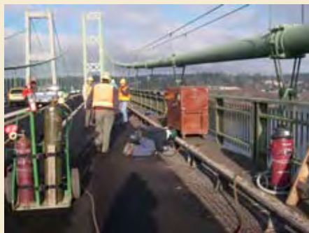
Crews remove the existing rub rail on the north side of the 1950 bridge.
