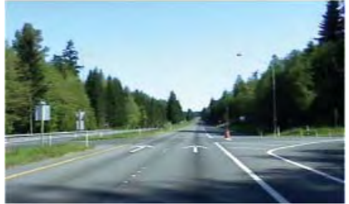
This safety improvement project on SR 16 channelized the intersection at Burley-Olalla Road to limit crossing and turning movements and added an acceleration lane
