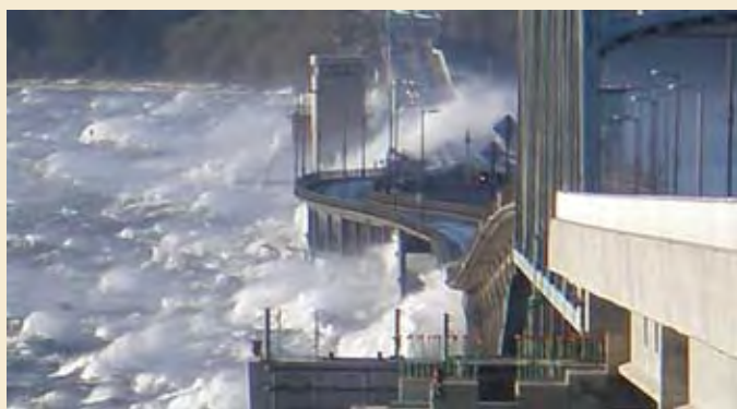
Hood Canal Bridge weathers a storm, October 18, 2007.
