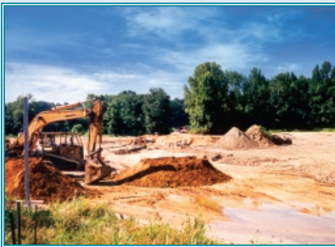
Grading a wetland restoration site, The Louis Berger Group
