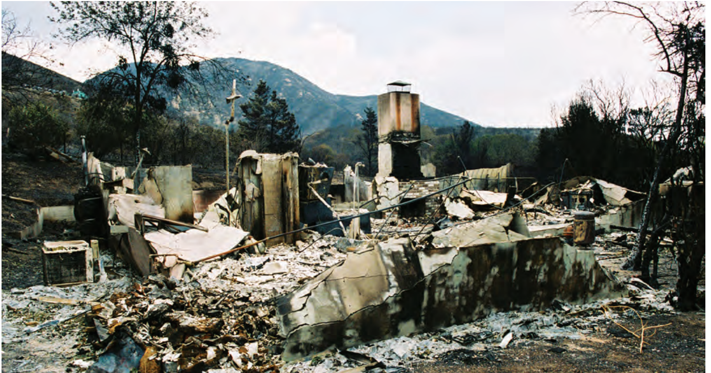
A wildfire left very little of this home near San Bernadino, California, in October 2003. FEMA photograph by Kevin Galvin.
