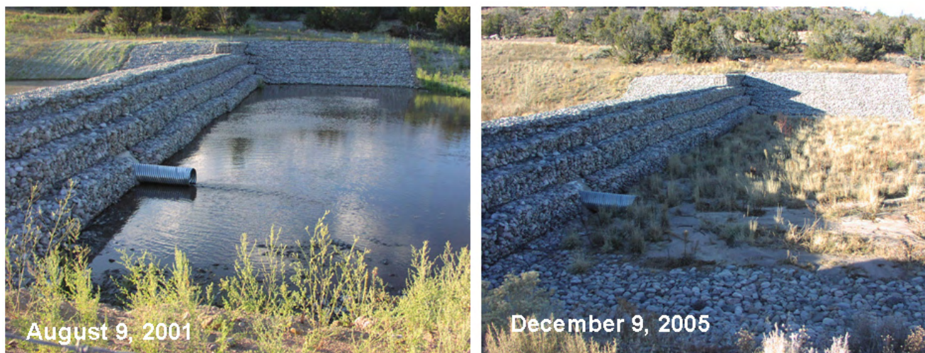
Figure 6-14. Low-head weir in Los Alamos Canyon retaining storm runoff and sediment. Notice deposition of stream sediments in basin of weir. Photographs courtesy of UDSA Forest Service.
