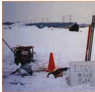
Site assessment equipment during the environmental studies along the I-355 extension route from I-55 to I-20.
