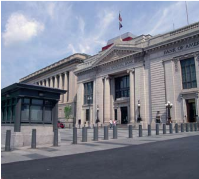
Address security needs: Washington, D.C. faces one of the greatest challenges in the nation in regard to providing both public access and security in the post September 11, 2001, environment. Retractable bollards and guard kiosks were part of the designed response to increase security at the U.S. Treasury building on Pennsylvania Avenue adjacent to the White House. However, terrorism is only one of multiple risks historic structures face.
