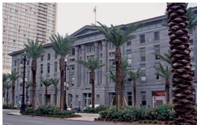
Parts of the U.S. Customs House on Canal Street in New Orleans, the Summit's venue, were constructed before the mid-19th century. Built as a symbol of the growing prosperity of the United States in one of its most important ports and centers of international trade, the cavernous and decorative Marble Hall was termed by one historic source "the finest business room in the world" at the beginning of the 20th century.
