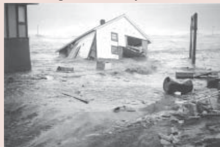
Wave erosion washes foundation away in Barrow, AK. Photo courtesy of Grace Redding
