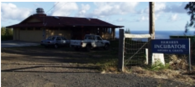
One of Hawaii’s shared-use kitchens.
