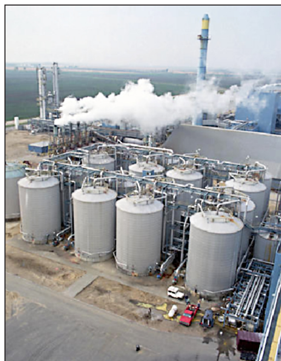
Ethanol plant. Photo: Warren Gretz.
