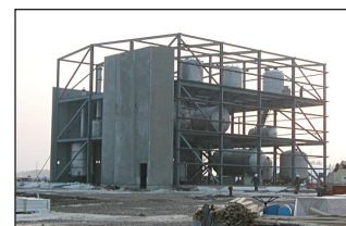
SoyMor Biodiesel plant under construction. Photo: SoyMor Biodiesel.
