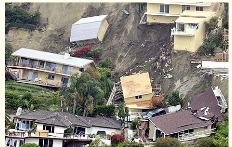
In June 2005, these homes in Laguna Beach, Calif., were heavily damaged during landslides triggered by record rainfall. (Photo by the USGS)
