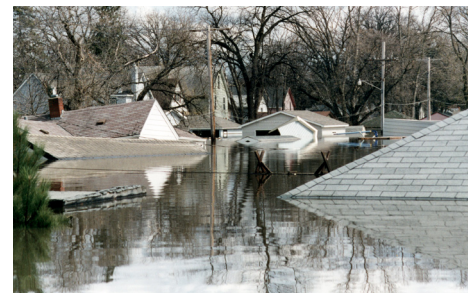
Homes in East Grand Forks, Minn., are submerged following flooding in 1997. (Photo by David Saville, FEMA)
